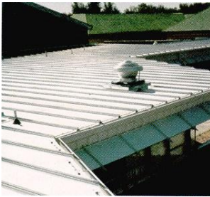
Bare standing seam roof
